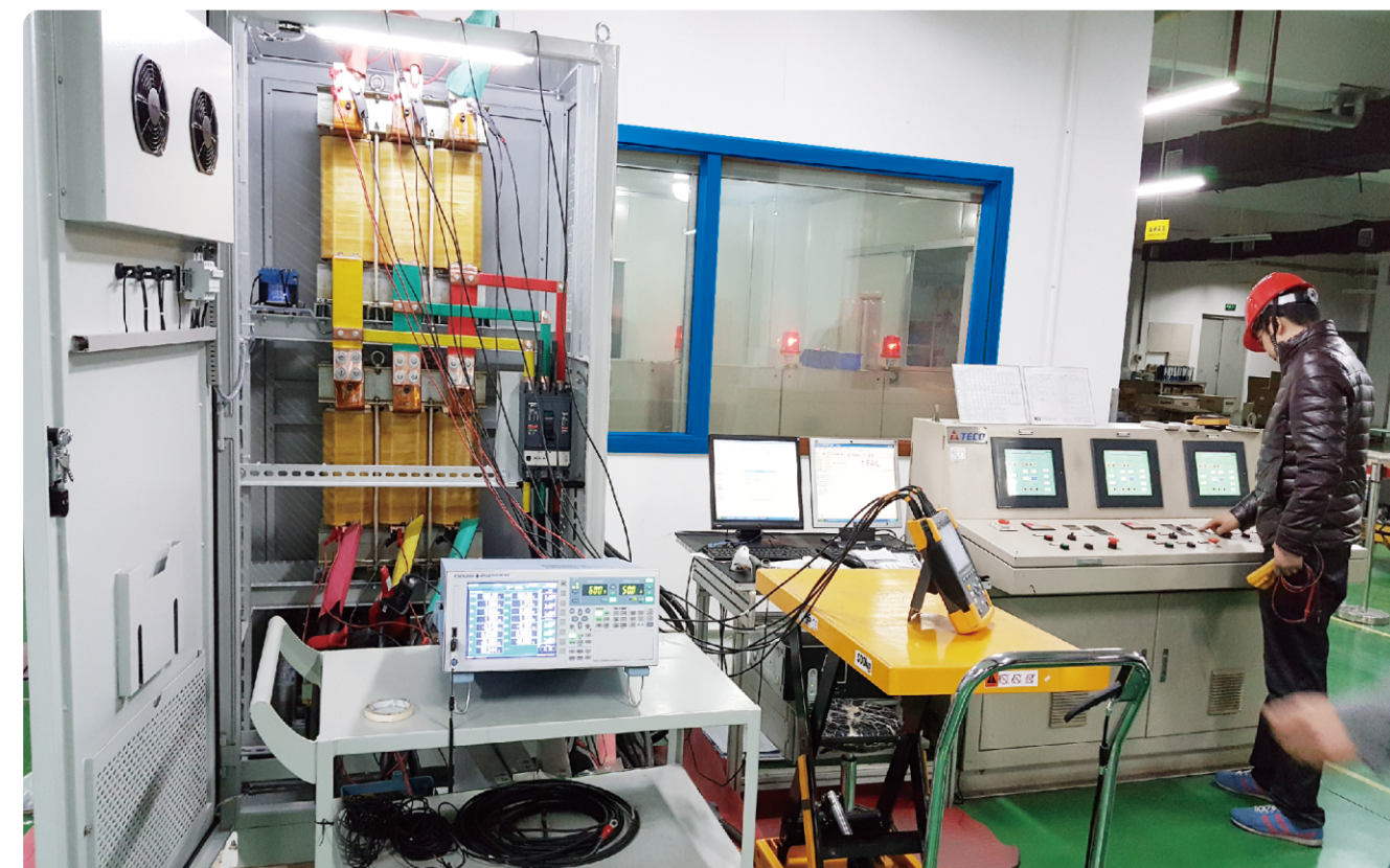
Passive harmonic filter performance testing
